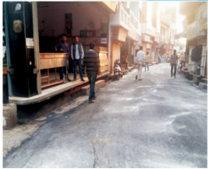
After Relaying: Chauk Bazar Kankhal to Anandmai Ashram Road, Haridwar, Defects removed
