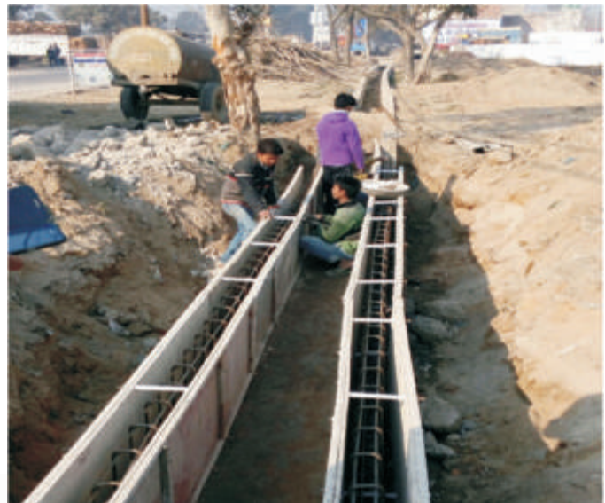
Reconstruction of dismantled Drainage work at Bahadrabad -Gagalhedi Road
