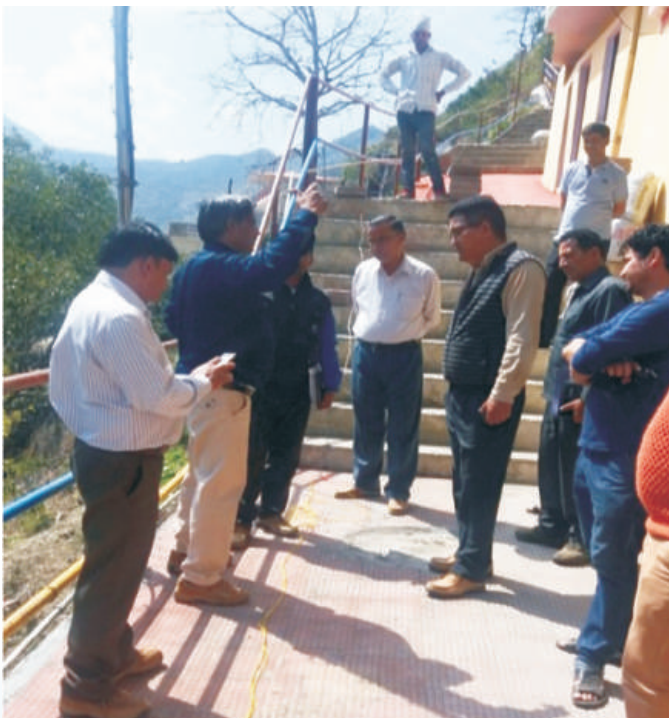
IRI Research Team found poor quality of Chequered Tiles in foot path in inspection with working agency, contractor, Rep. of Chairman & SDM Kritinagar of Nagar Panchayat, Devprayag work under AKM-2016
