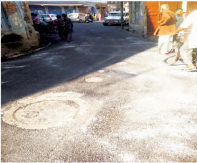
Before Relaying: Pot holes found on Chauk Bazar Kankhal to Anandmai Ashram Road, Haridwar.
