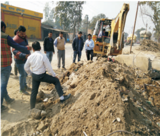
Dismantling of poor quality Drainage work at Bahadrabad -Gagalhedi Road
