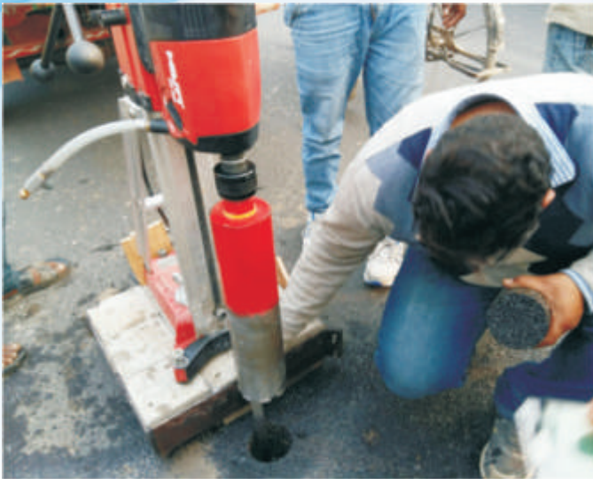
Quality Control & Assurance work by Irrigation Research Institute, Roorkee under AKM-2016
