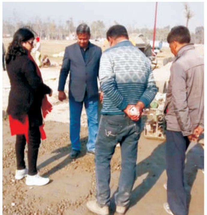
IRI Research Team observed the deficiency in CC Road construction works at Pant Dweep in presence of Secretary, HRDA, Haridwar work under AKM-2016
